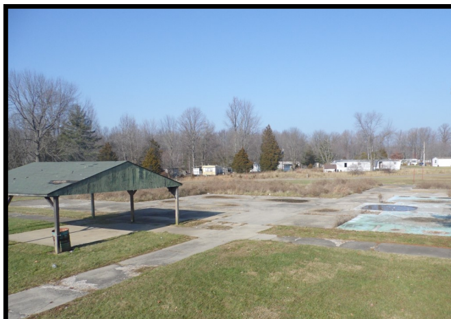
Abandoned pool near playground at CSL
