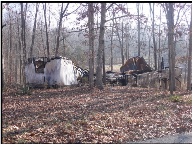
Damaged home structure at CSL
