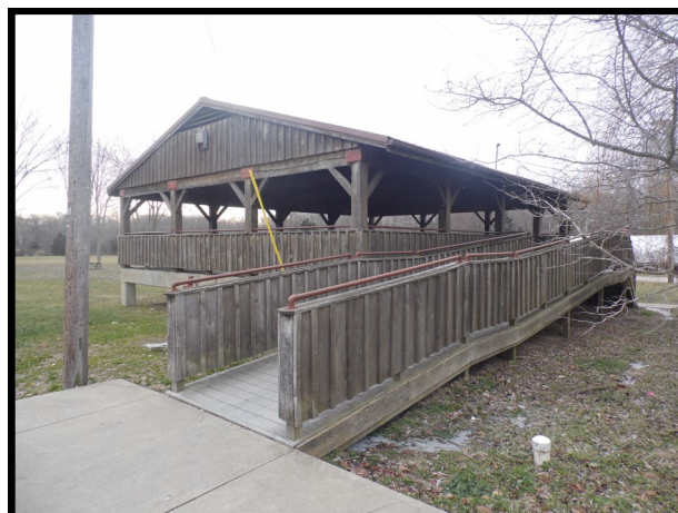
Long wooden ramp to the raised shelter at the Muscatatuck Park.
